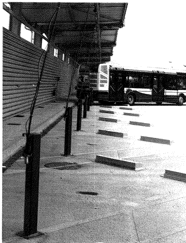
Fig. 2-7: Slow-filling station in Poitiers, France
